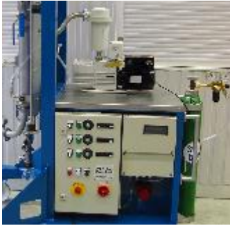
Figure 12: electrical control unit of TGD20a and GKM15a
