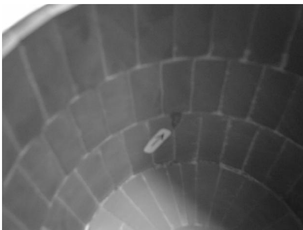
Figure 13: one of two cracks in the lining plates, both appeared in cylinder-lining
