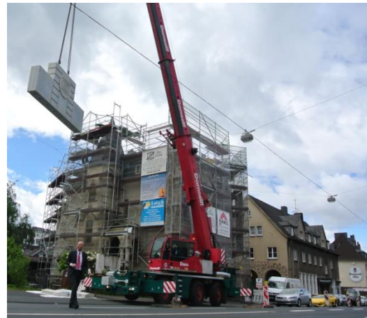
roof balustrade at “Villa ZCS”: 6 x 6 meter, 12 tons FuturBeton
