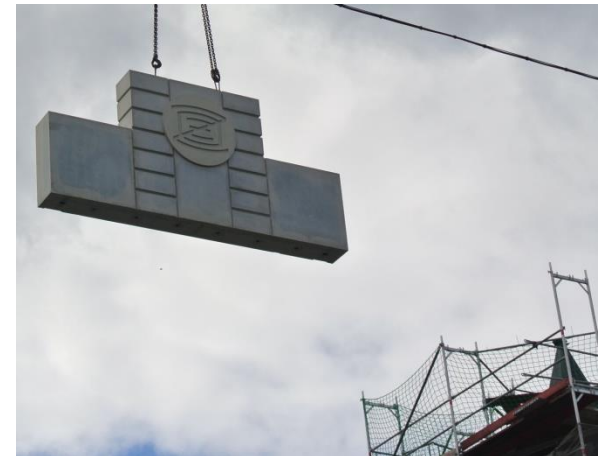
roof balustrade at “Villa ZCS”: 6 x 6 meter, 12 tons FuturBeton
