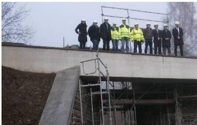
Fig. 7. Bridge Rosenthal at Olpe/Germany
